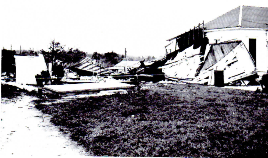
FIGURE 4.—Complete destruction of wooden house constructed with no studs in the outside walls. Undamaged house next door was of approximately the same age.
